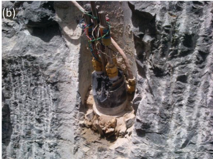
Figure 3. (a) Anchor displacement of a damaged MPBX (b) Photograph of the head of a damaged MPBX).
